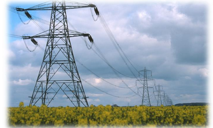
Transmission Line Project
